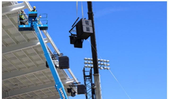
Sound Image specified six clusters, each consisting of one QX594i to cover the near-and mid-field, and a QX596i for long throw. The QX594i's 90x45 dispersion covers a wide, but controlled, sector, while the 60x45 dispersion of the QX596i provides far-field coverage.
