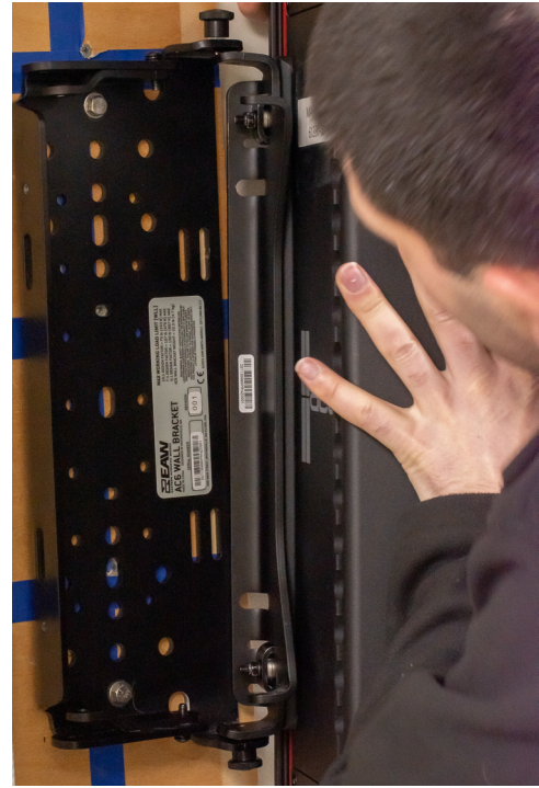
Attaching AC6 to wall bracket
