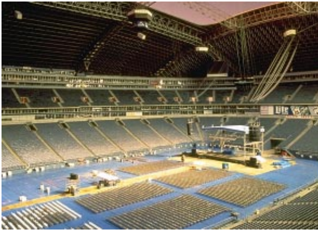
KF853's, KF852's, BH852's and KF850E's arrayed for the Promise Keepers at Texas Stadium – where RT 60 's are in the 10 second range – by Spectrum Sound of Nashville.
